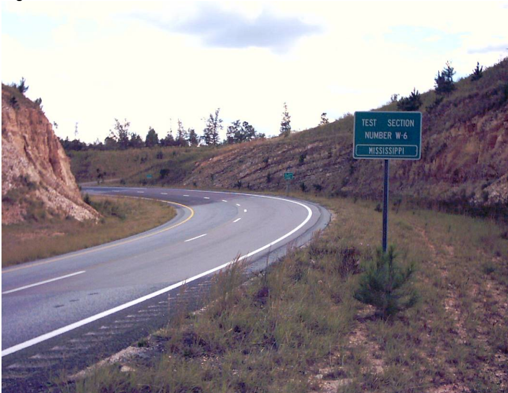
Figure 2 Mississippi 4.75 mm HMA Section W6
